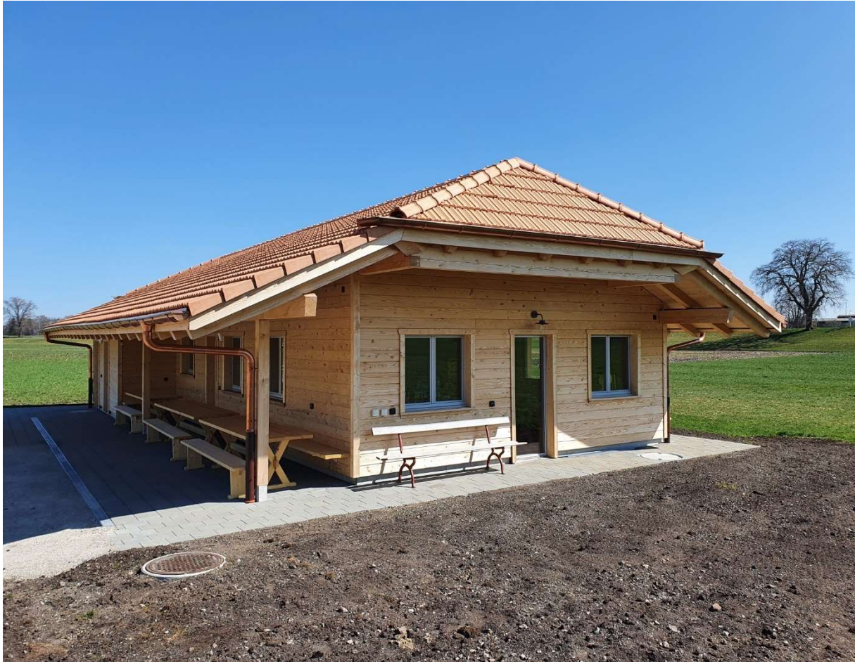
Abb. 2: Neubau Clubhaus (April 2021)
